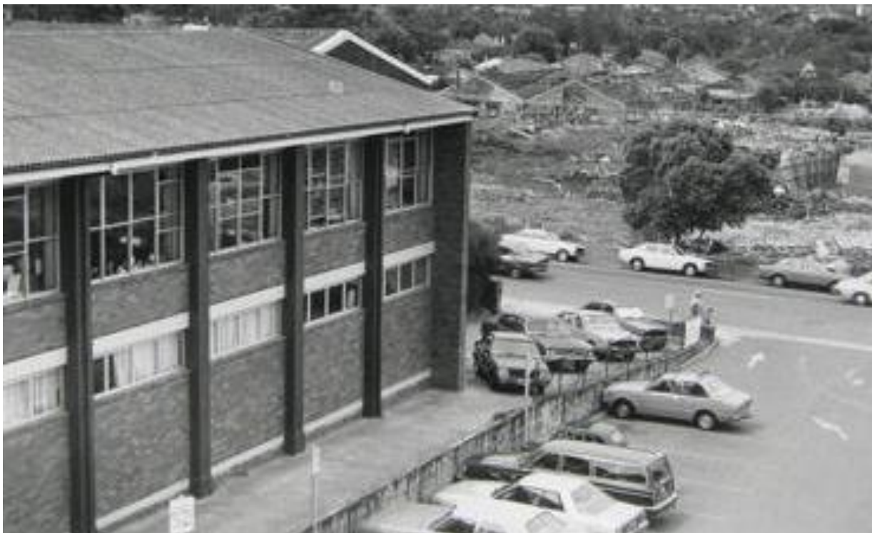
Picture 11 – Former Willoughby Municipal Council Depot prior to its demolition for Chatswood Chase.
