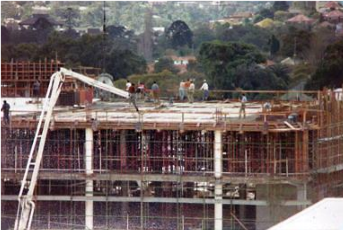
Picture 12 – Chatswood Chase under construction.
